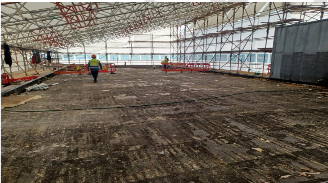
Images above: progress on Town Centre House
